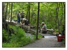
The boardwalk that runs along the west side of Pine Knob's Meteer Lake was replaced. Approximately 900' of new treated lumber boardwalk was constructed.
